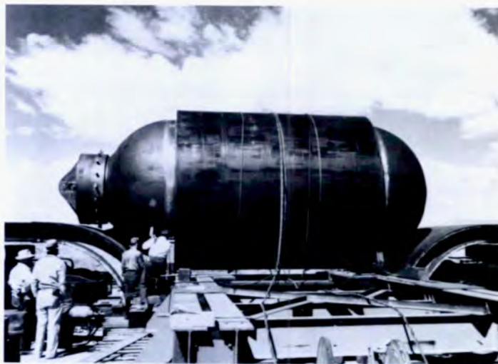
Jumbo was designed to withstand the explosion of HE and permit recovery of active material should the Trinity shot fail. It was not used.
